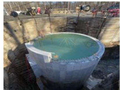
MH31 Leak Test
