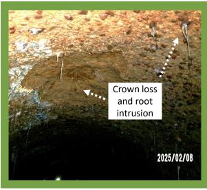
**PROJECT SPOTLIGHT:** Recent EWOS & EWORS inspections identified areas with significant wall loss. Emergency bypass channel for EWORS constructed and rehab forecasted for completion by November. Additional rehab planned under PDB contract.
