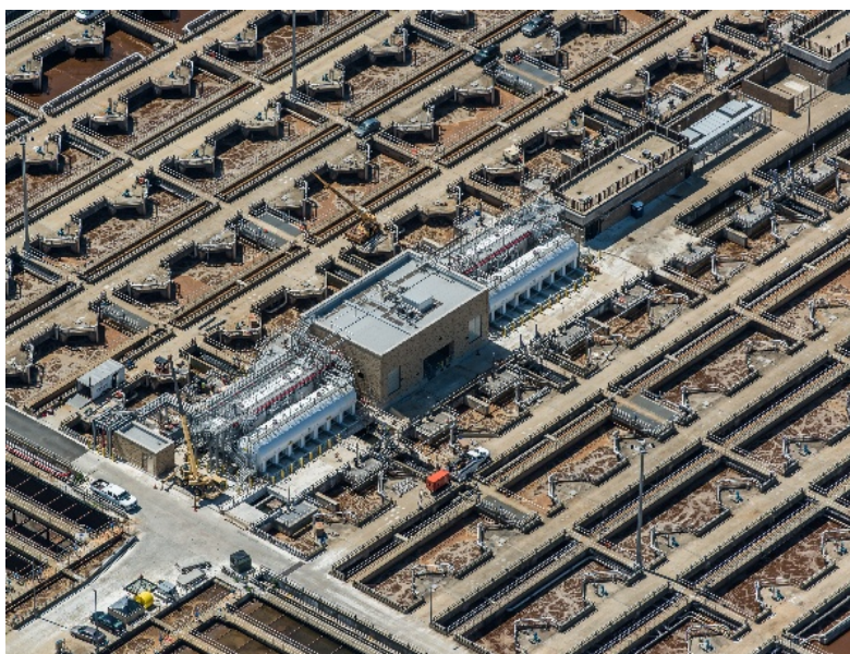
Aerial view of Wastewater Treatment Plant
