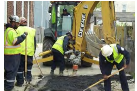
Linear Pipe Restoration
