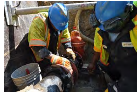
Water Meter Installation
